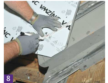
8 Roof panel measured for cutting.
