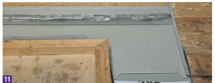
10 Back plate with soldered strip.
