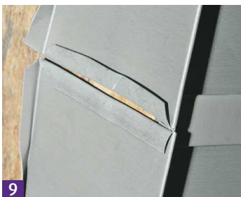
9 Fit adjoining flashing and turn up folds.
