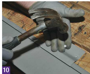
10 The eaves strip must be installed with a zinc cleat.
