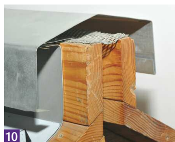
10 Insert ridge flashing.
