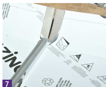
7 Seam panels together.
