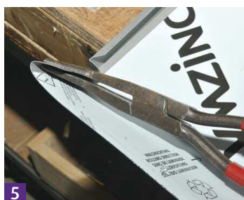
5 Create fold on panel upstand.
