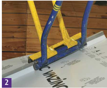
2 The seams are crimped beyond the hip.
