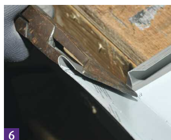
6 Finish fold on panel upstand.
