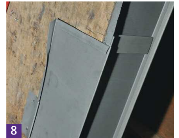
8 Fit fascia with a cleat.
