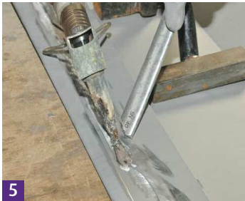
5 After applying flux, solder the cleat to the valley.
