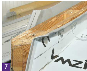
7 The hip batten is installed.
