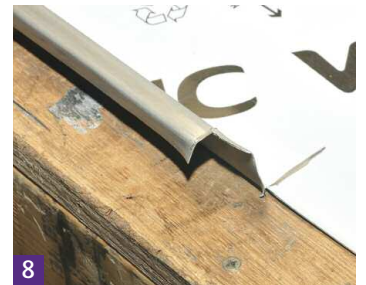
4 Create dog ear fold at bottom of rooflight.
