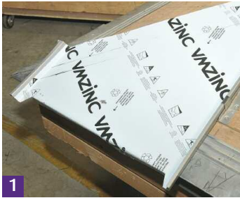
1 Panels are installed on the hip.
