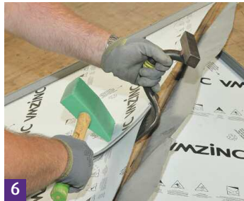
6 The seams are again flattened.
