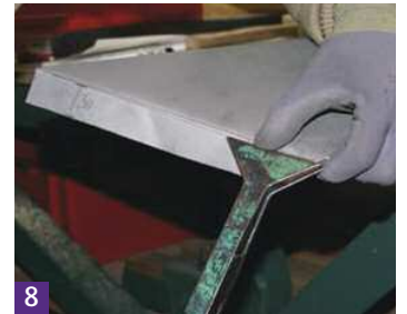
8 The end of the G3 hip is folded back over 30mm.
