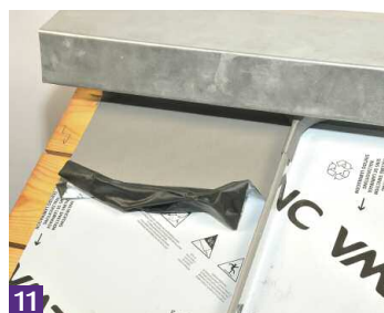
11 Do not partially remove film.
