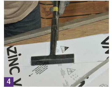
4 The panel is folded upwards.
