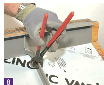
8 Fit saddle piece and pinch at seam.
