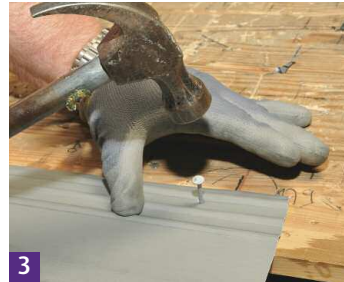
2 The G3 eaves strip located in position.
