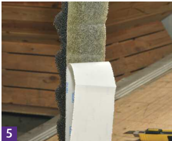
5 The tape is removed from the compression strip.
