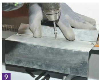
9 Fit clip for ridge flashing.
