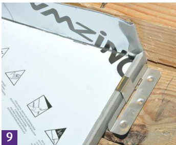
10 Peel back film on area to be soldered.
