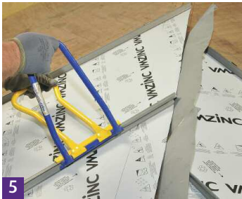
5 Panels on the other side of the hip are seamed up.
