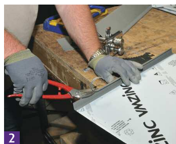
2 Cut away return fold on the profiles.
