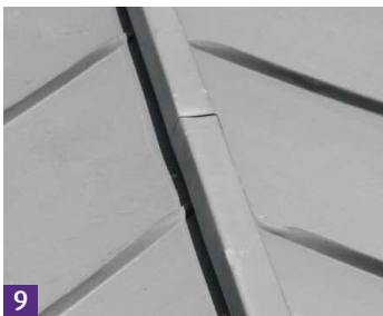
9 The completed hip
