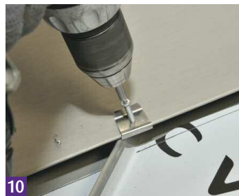
10 The G3 hip is installed into the clip and fixed with a stainless steel screw.
