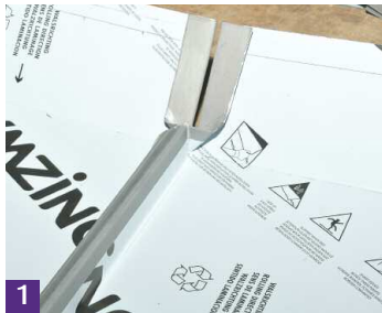
2 Pinch saddle piece into place.
