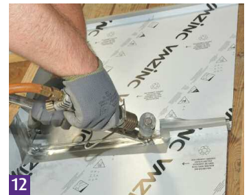
8 Cut back standing seam by 25mm. This enables a tab to be folded back prior to soldering above the rooflight.
