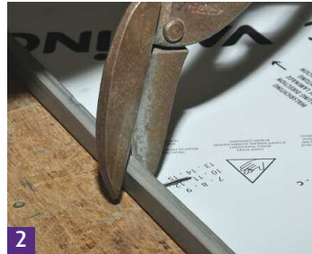
3 Fold back standing seam.
