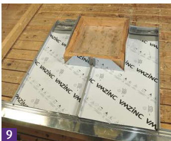
10 Back plate with soldered strip.
