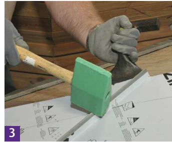
3 The seams are carefully flattened over 150mm.
