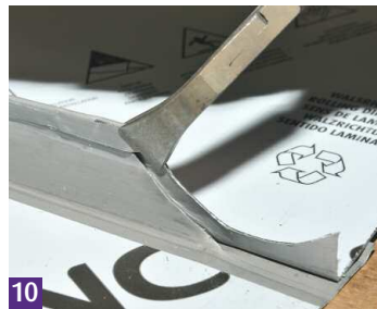
9 Cut the zinc back.
