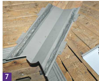
7 Valley ready to receive roofing panels.
