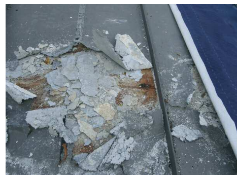
Result of using a hybrid roof.
