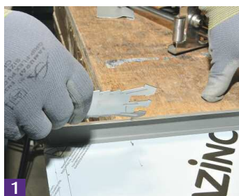
1 Mark the zinc at 100mm.
