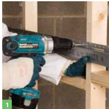
2 Resilient Bar fixed to one side
