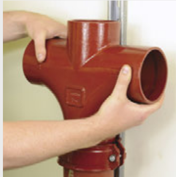
3. Push the second pipe or fitting into the coupling again ensuring that the spigot is abutted against the central register.
