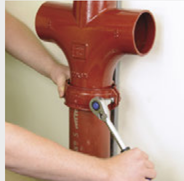
4. Check alignment of assembly before tightening the bolts. Coupling bolts on all sizes are M8 and require special Allen socket adaptor (6mm) EF102, together with a ratchet spanner EF100. Alternatively use a time saving power tool.
