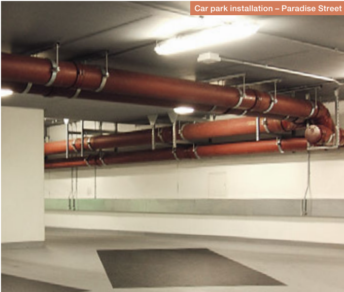
Car park installation – Paradise Street
