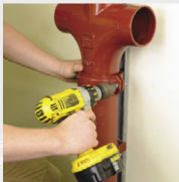
3. Push the second pipe or fitting into the coupling again ensuring that the spigot is abutted against the central register.
