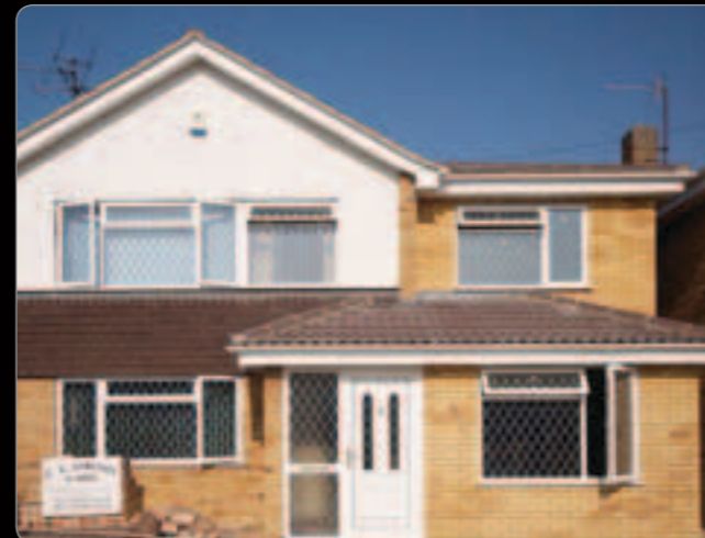
Golden Buff - Example of an extension matching London bricks to existing ones
