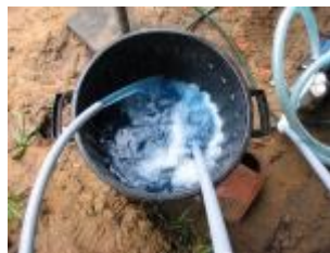
Fig 40 Purging the Slinky of Air
